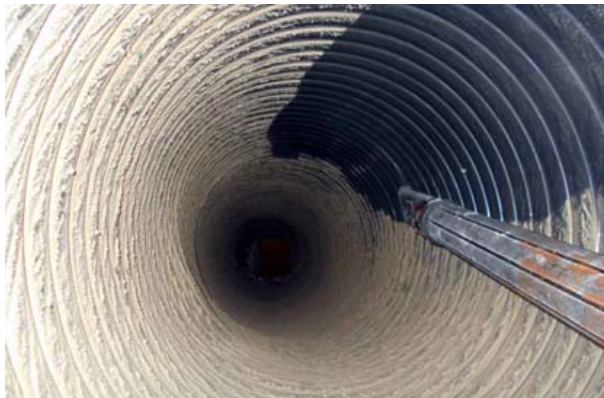
Dust in AC ducting always harbors not only mold but dust mites, bacteria and viruses. Must restore to "as new" clean for sensitive people.
